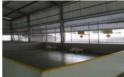
Abu Kerak Boiler, Boiler, Fly Ash Insinerator
