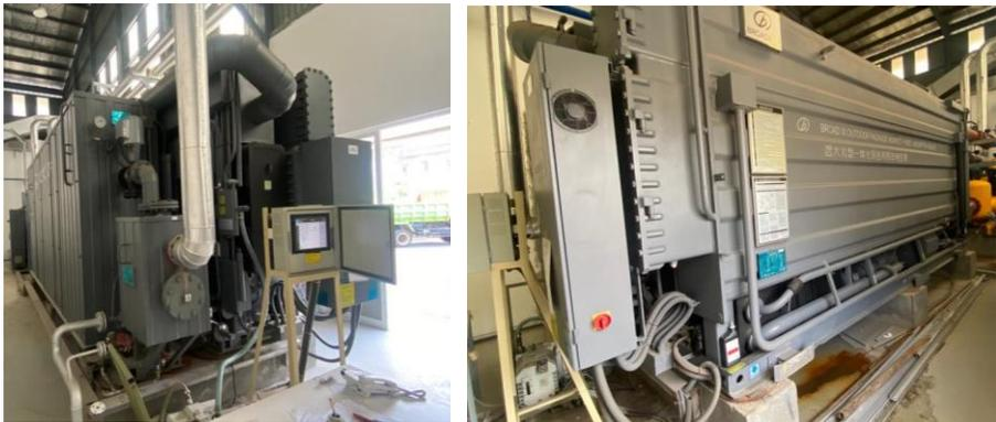
**Gambar 4.3. Absorption Chiller di Unit RTD**
