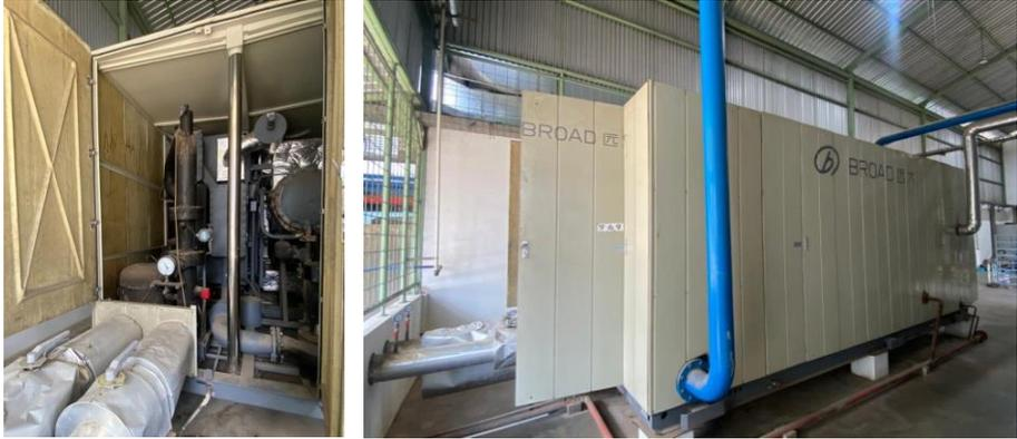
**Gambar 4.2. Absorption Chiller di Unit Pil Jamu**
